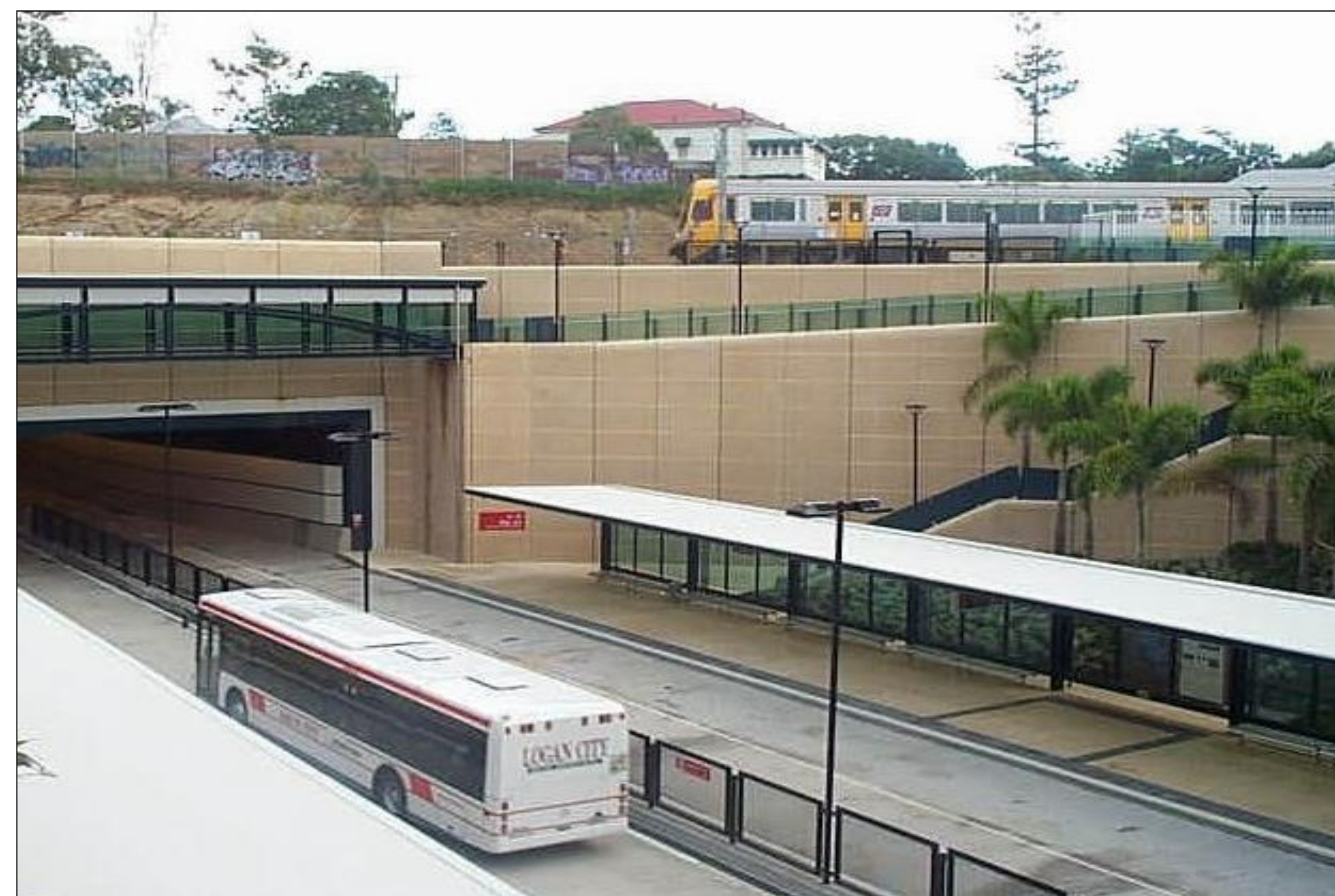
Example of a BRT System
